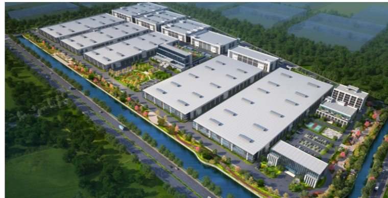
📍 Huzhou Manufacturing Headquarters
